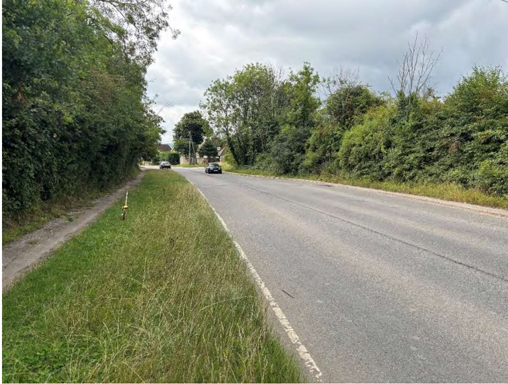
Site 1 - Photo 1 - view looking south along South Road towards junction of Mill Lane
