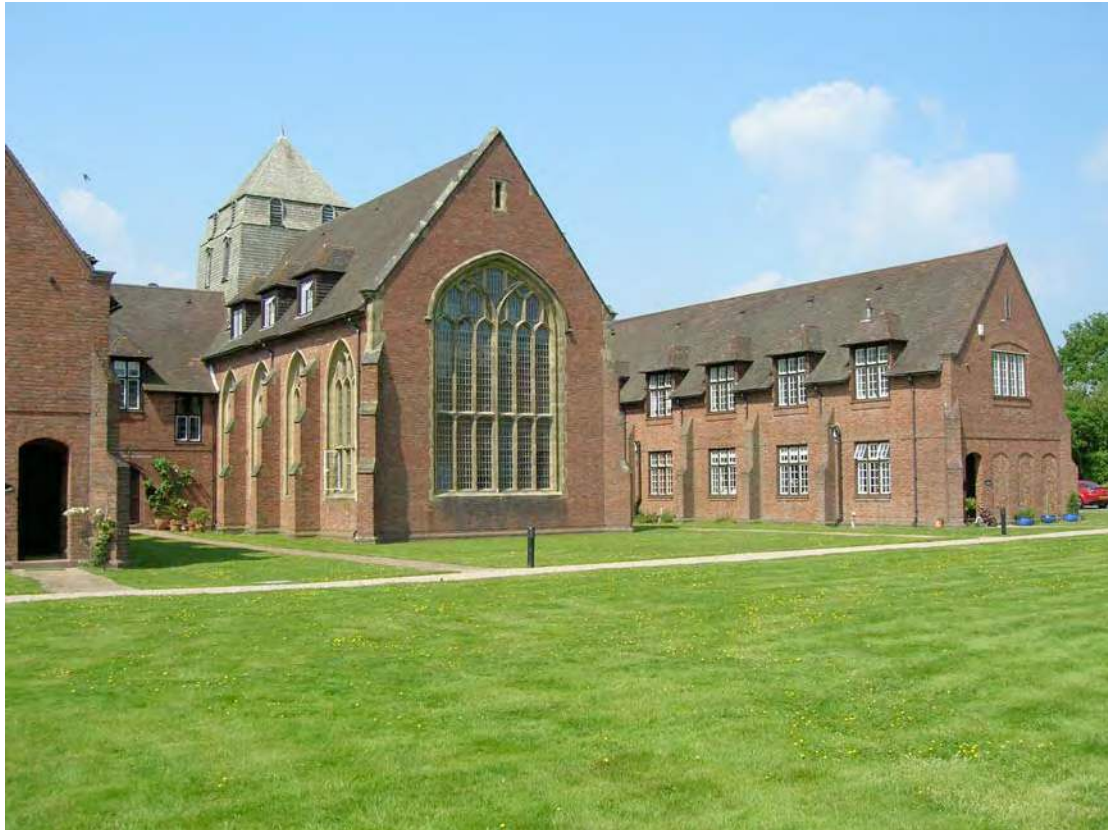
South elevation of St Georges
